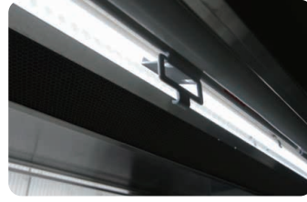
LED 조명 LED lighting
